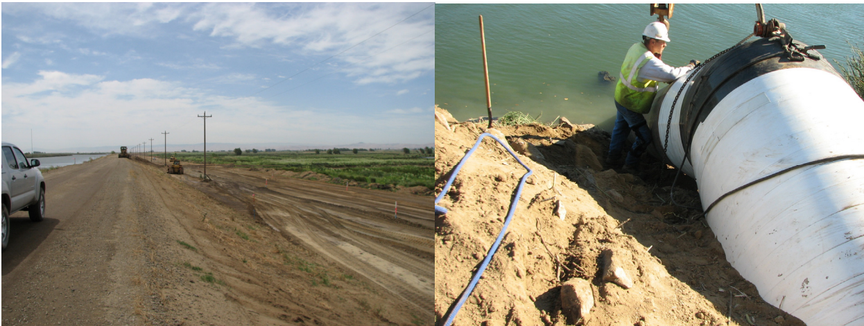
Photos of levee repair and a pipe replacement by MBK Engineers.
